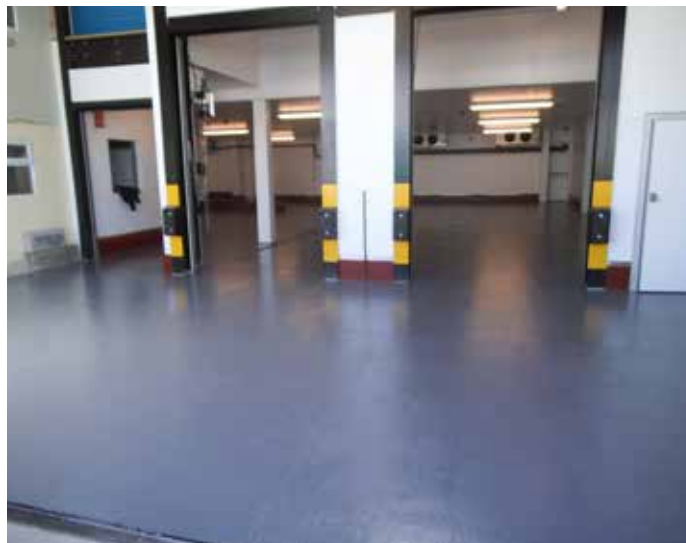
Dairy warehouse floor restored with Belzona 5231
