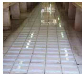
Tiled floor after
