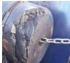
Damaged part rebuilt
