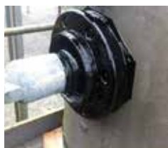
Transformer leak sealing
