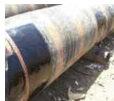
Floating hose repair
