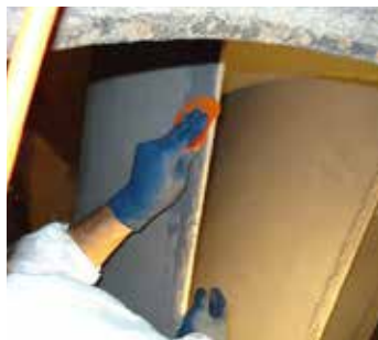
Forming and rebuilding
