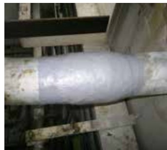
Wrapping and patching
